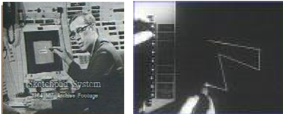
Figure 5: Ivan Sutherland at the console of the TX-2 using his Sketchpad System at Lincoln Labs, MIT, 1963. He is holding a lightpen in his right hand, which he used to interact directly with the screen. The right hand image is a close-up of the lightpen being used for graphical input.
